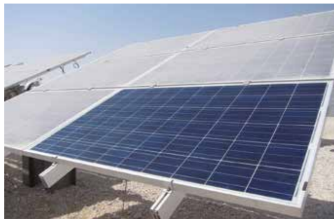
The soiling of solar modules with sand and dust reduces output in desert regions.
