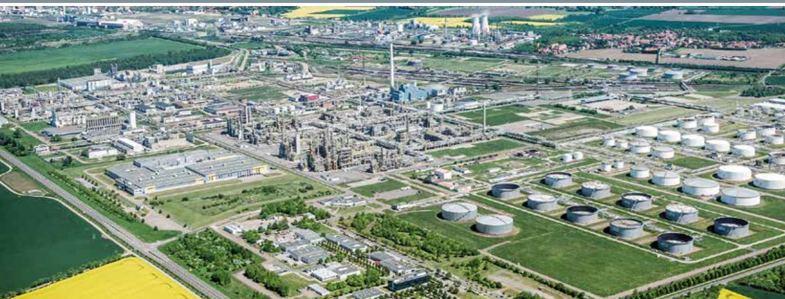
25 | In the future, large-scale water electrolysis at the Leuna Chemical Complex will provide sustainable support to the chemical industry.
