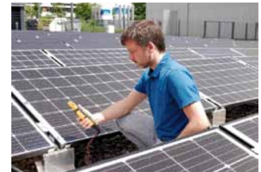
By using the electricity generated by the solar plant at Fraunhofer CSP, around 37.5 tons of CO 2 could be saved in 2021.
