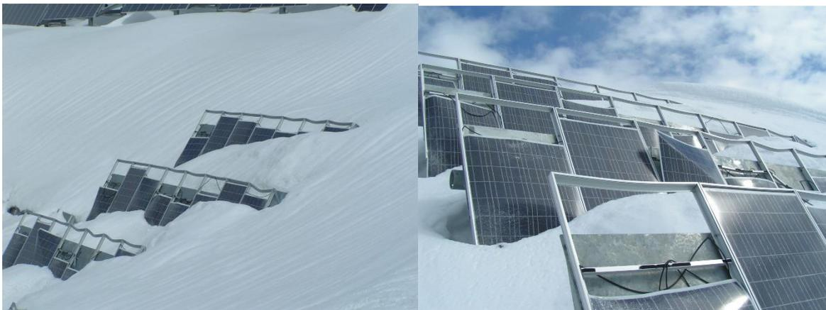
**Figure 16: PV-system at Wildkogel/Austria; wrong site-selection: every winter, a snow roll always covers the PV fields and causes severe damage; the PV plant must be relocated.**
