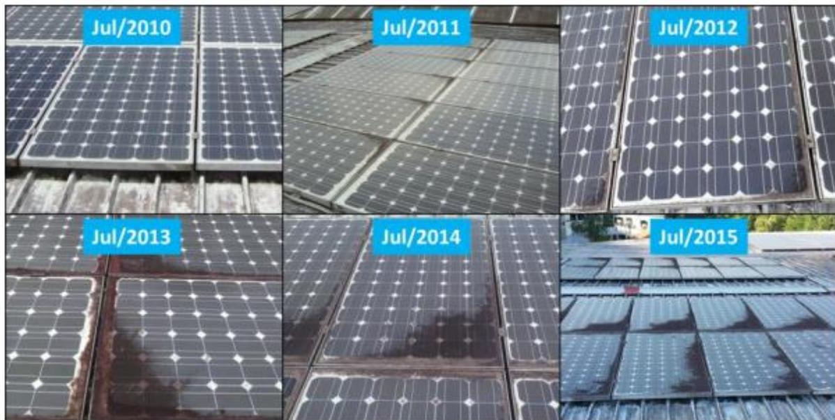
**Figure 37: Evolution of soiling on an unmaintained flat PV system in Singapore [216].**
